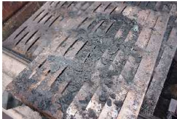
Remove and clean Heat Plates
