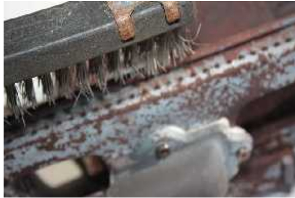
Burner brushed down and partially cleaned.
