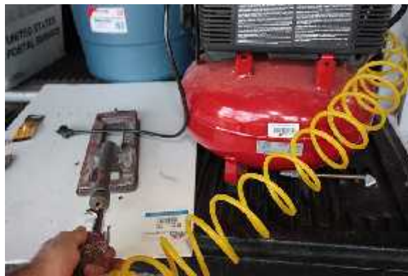
Blow out the burner through venturi opening with compressed air.
