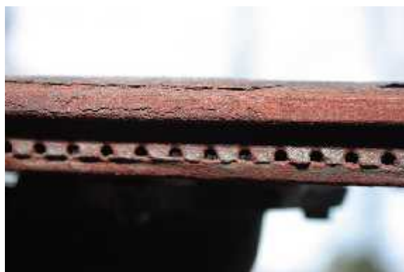
Blow gas ports with compressed air.
