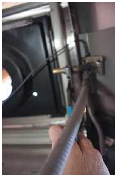
Loosen side burner on orifice with wrench or channel locks.
